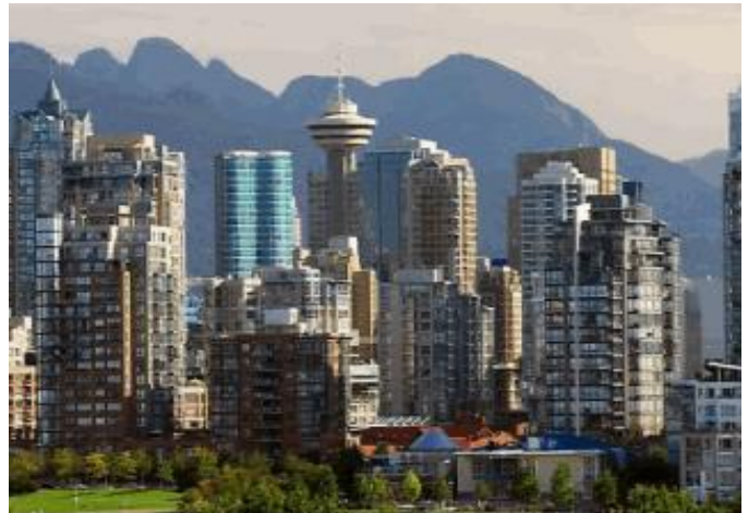
View looking North
